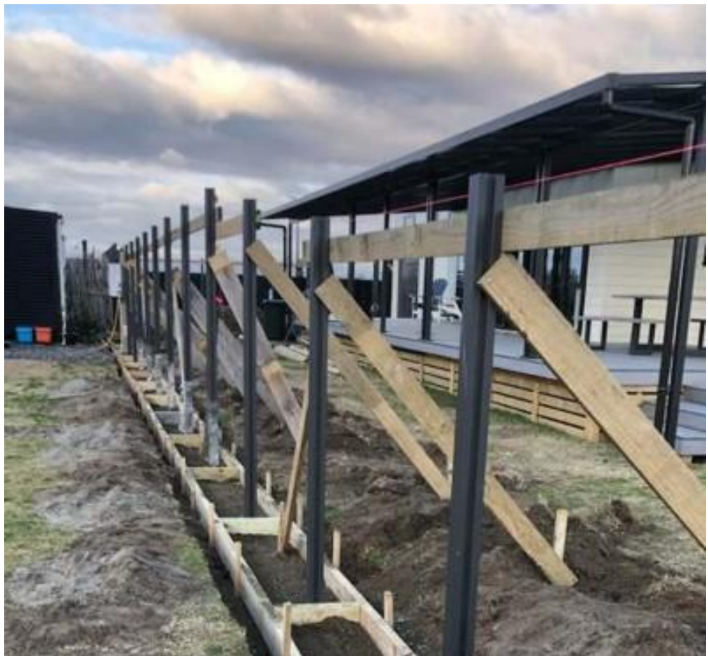
3B-E. Concrete posts in place
